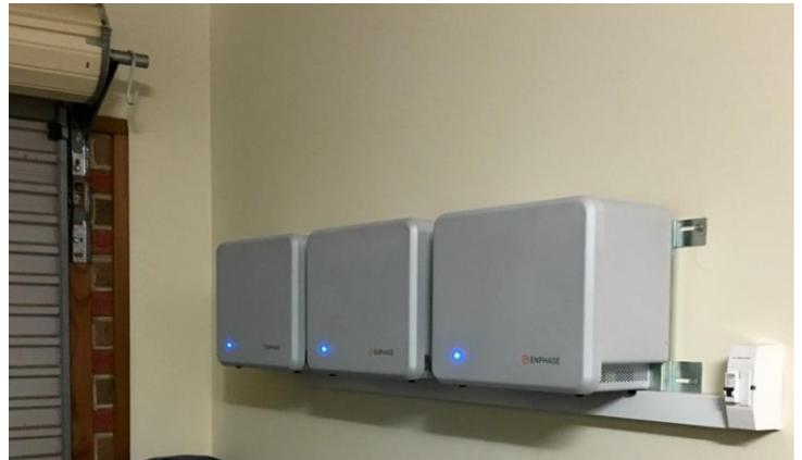
The Enphase batteries are not rated for outdoor installation so must be installed indoors in a non-habitable room e.g., garage, hallway, weatherproof porch, laundry. The Storion inverter and the Selectronic SP Pro hybrid inverter and BYD batteries can be installed outside in a location away from the sun—although we always recommend an indoor location if possible.
