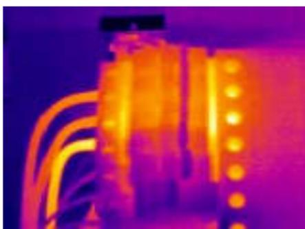
Most electrical or mechanical parts that are damaged or ready to fail will generate heat. The camera will detect this heat and show it in graphic form. After capturing images of your systems we then prepare a written report showing which
